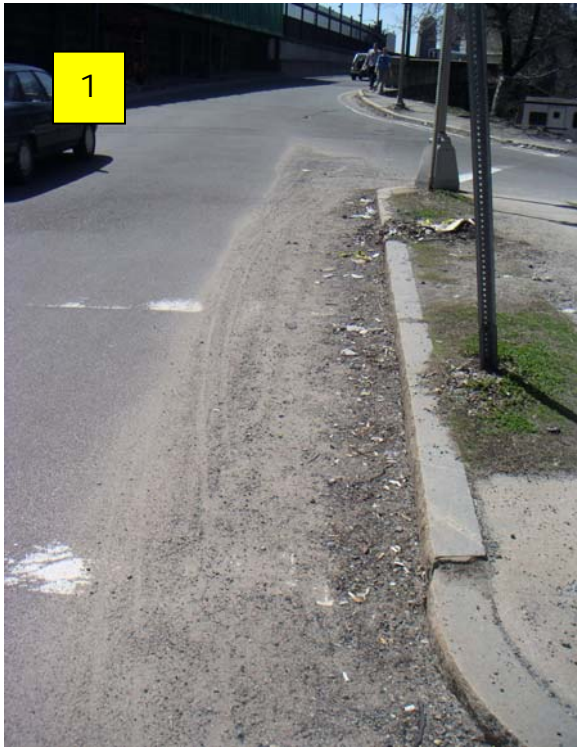
LONGFELLOW BRIDGE: WESTBOUND
